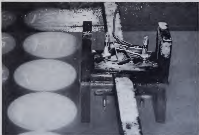
Figure 65.—A view of thermoregulators in a curing water tank. P126-D-75009.
